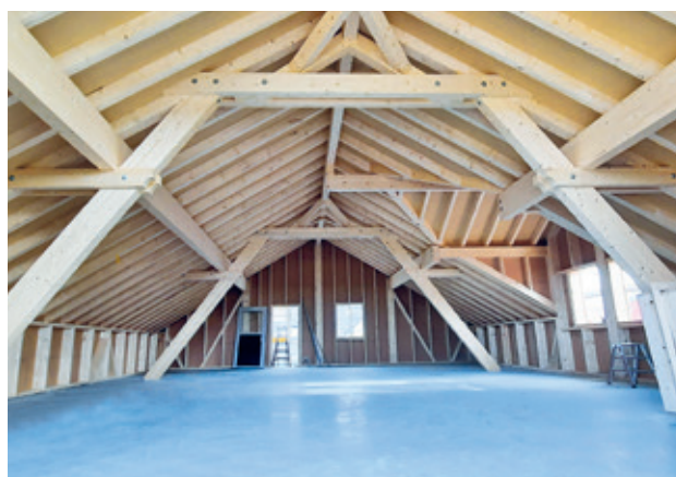
Visible framework in residential home, Rothenburg (CH)
