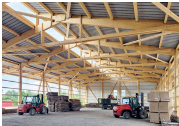
Industrial hall, Bartenheim (F)
